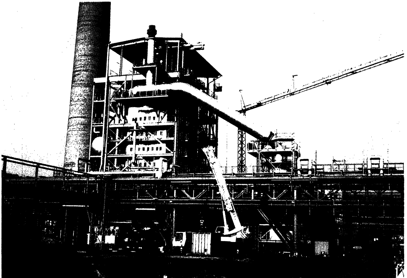
Construction of a flue-gas cleaning plant: BASF, Schwarzheide (Land of Brandenburg, Germany)
