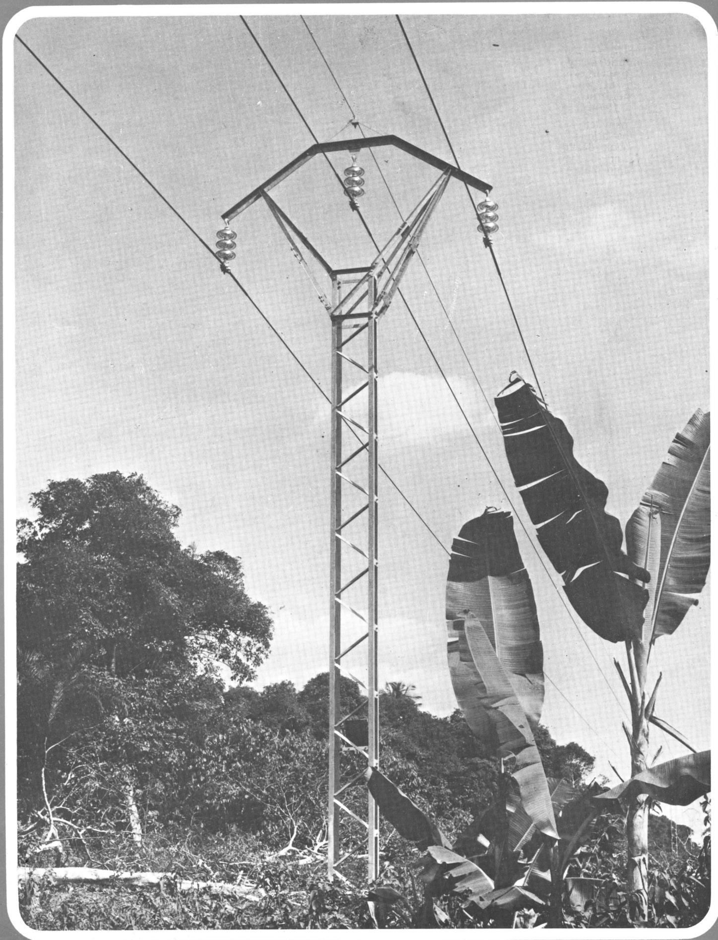
*High tension (33 000 volts) transmission lines serving the region around Lagos (Nigeria)*
