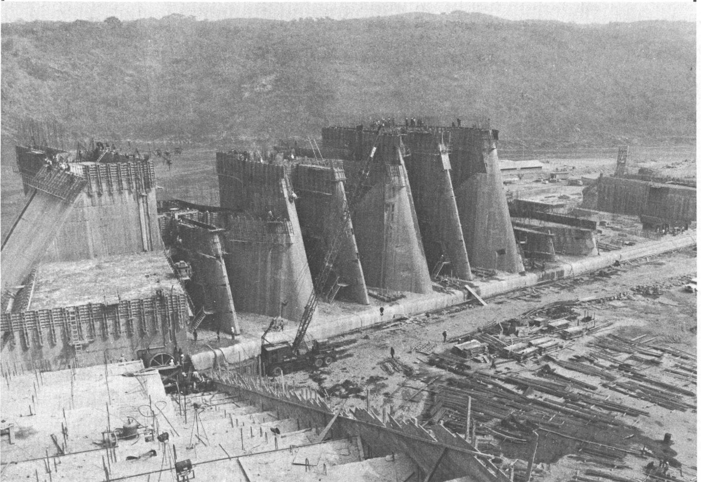
*Building part of the Inga dam on the Zaïre river. This single hydroelectric complex has the potential to produce nearly a third of the world's hydroelectricity.*
