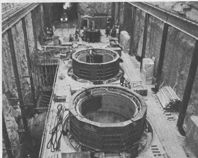
*Hydroelectric power station at Kamburu (Kenya). Each of the turbine generators has a capacity of 130 MW.*
