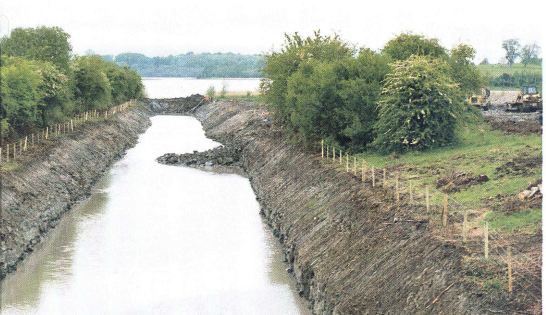
The Ballinamore - Ballyconnell Canal: A major cross - border project funded under INTERREG.
