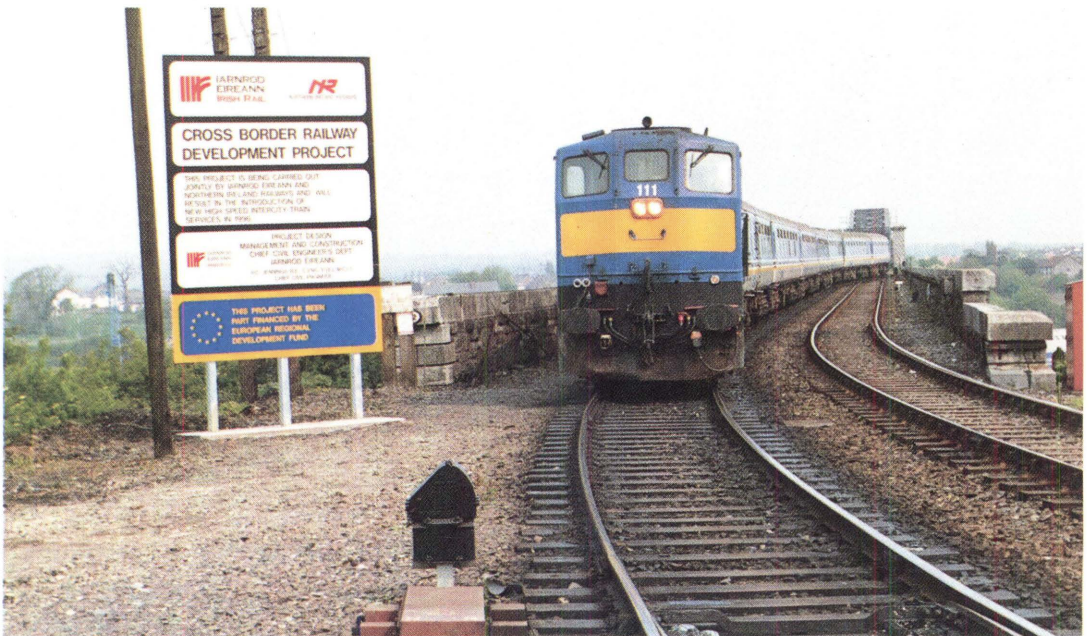
The Dublin - Belfast Railway being upgraded under ERDF
